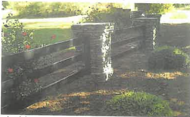
A similar example of the style of the craftsman fence of board and stacked stone that will complement the road frontage at Crooked Creek Road and Crooked Creek Drive.
