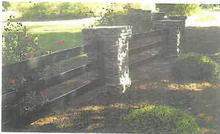
A similar example of the style of the craftsman fence of board and stacked stone that will complement the road frontage at Crooked Creek Road and Crooked Creek Drive.
